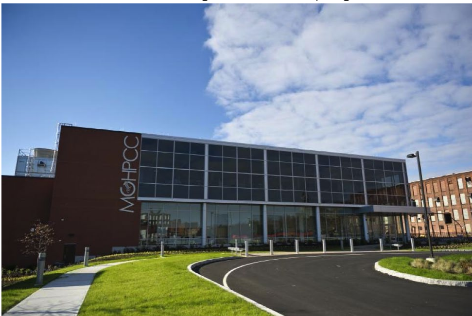
The Massachusetts Green High Performance Computing Center
