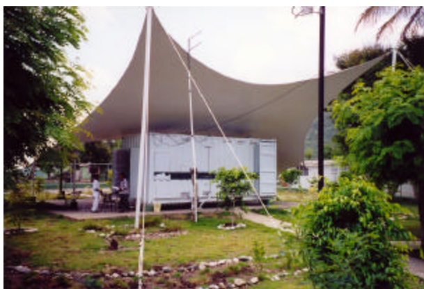
Figure 18: The first five LINCOS units used the recycled shipping container.
