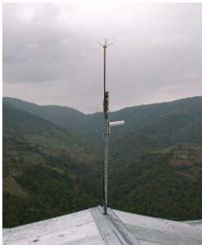
A customer premises antenna and call-processing unit. (Source: Bhutan Telecom)
